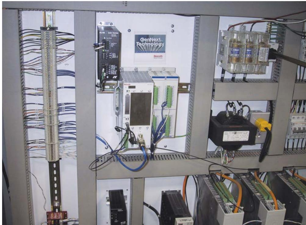
Spearheading the control package are the Bosch Rexroth PPC-R, a powerful controller in a small size, and the EcoDrive Cs drives which provide industry-standard interfaces including SERCOS, DeviceNet, CANopen or PROFIBUS-DP.
